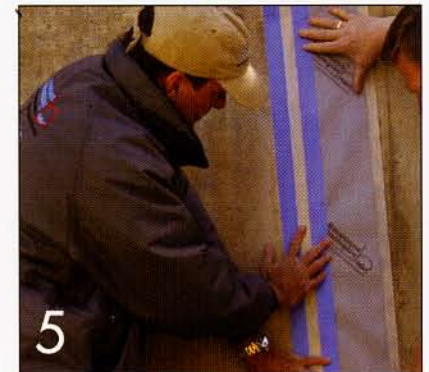
5 Finishing the Techni-Crack membrane with sealant
