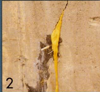
2 Optional polyurethane injection stops water from the outside of the wall (for really “bad” leaks).
