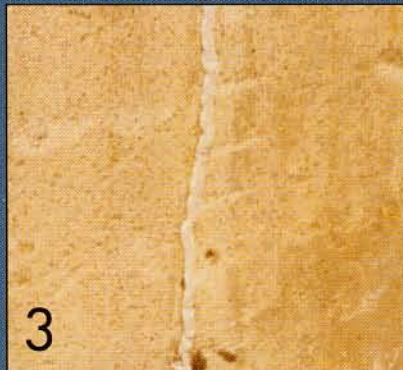
3 One part polyurethane sealant on the crack.
